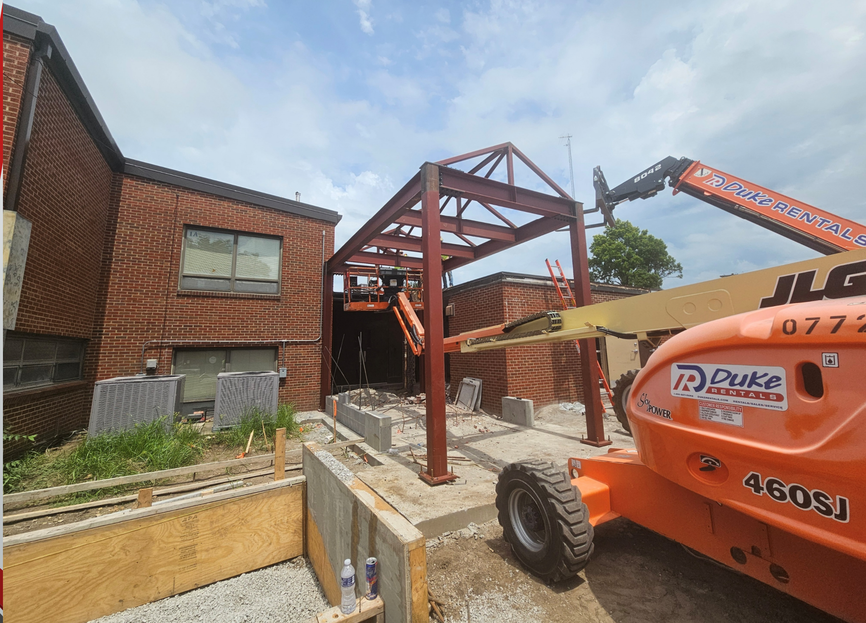
Structural Steel framing for new High School Entrance
